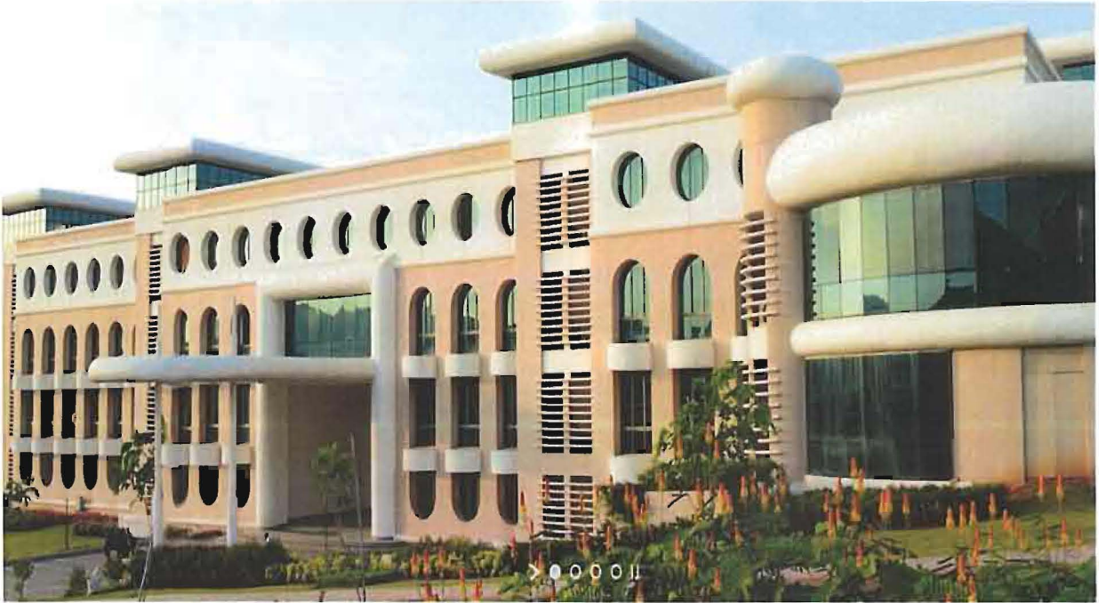
Photo No. 3: Building of Sandip Institute of Pharmaceutical Sciences
