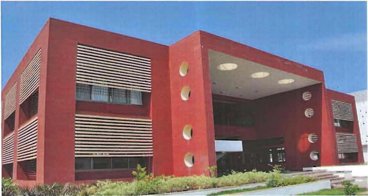
Photo No. 16: Library Building
