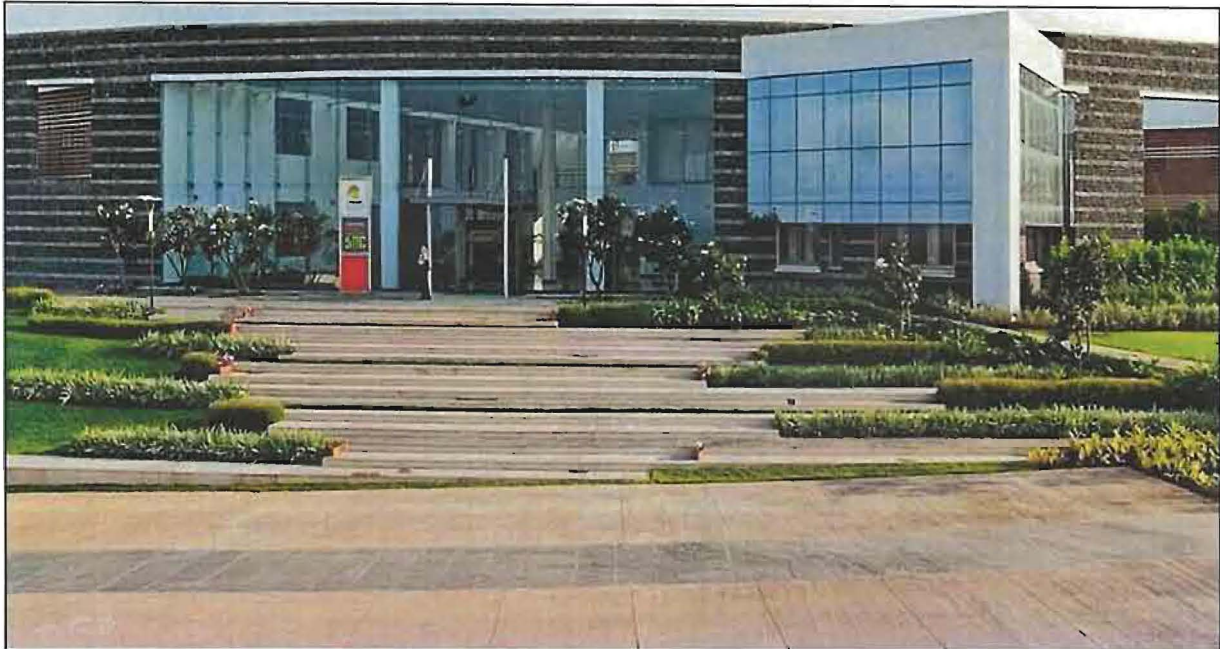
Photo No. 1: Building of Sandip Institute of Technology and Research Centre
