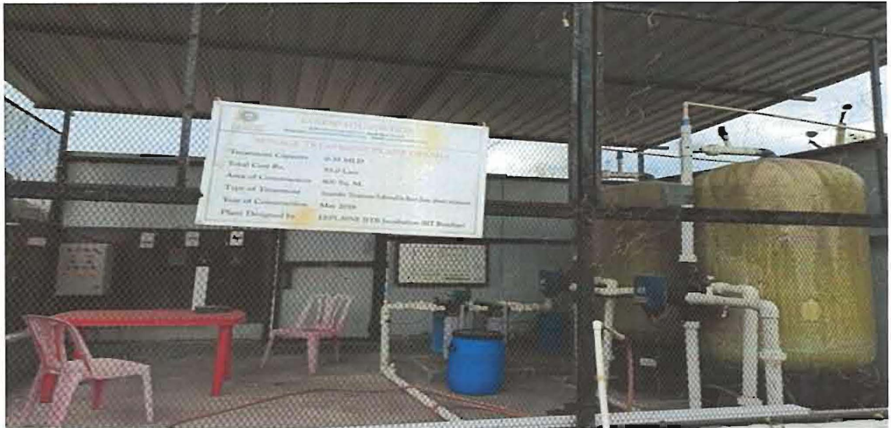
Photo No. 27: Sewage Treatment Plant Facility (A), (B)
