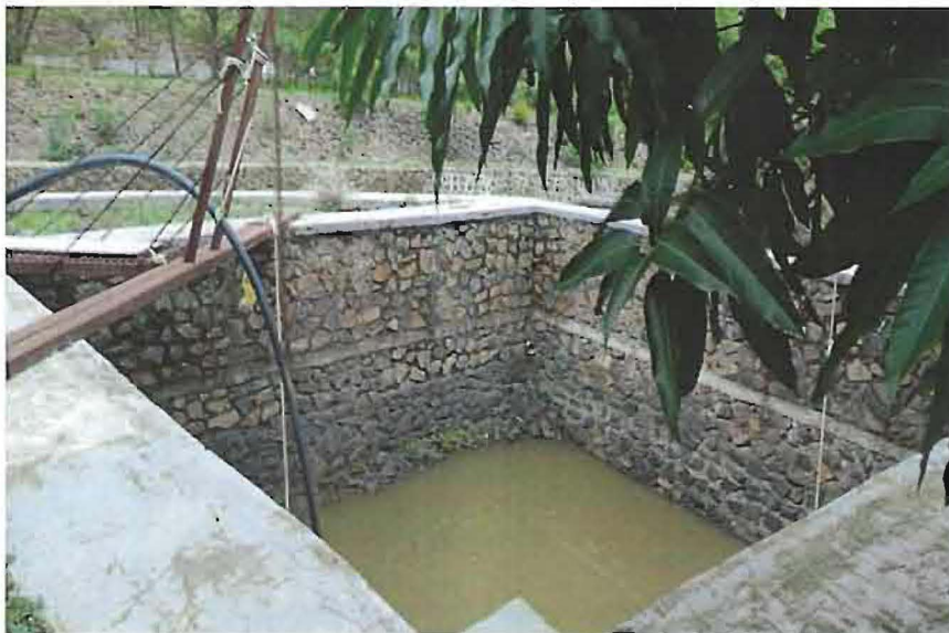
Photo No. 23: Storage tank facility
