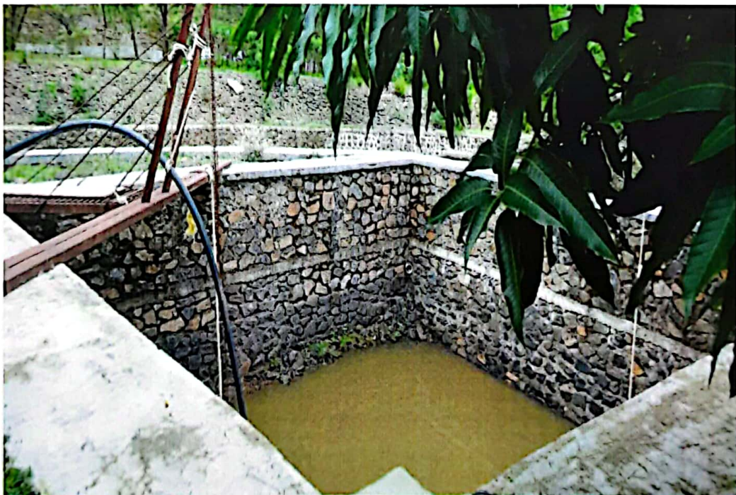
Photo No. 23: Storage tank facility
