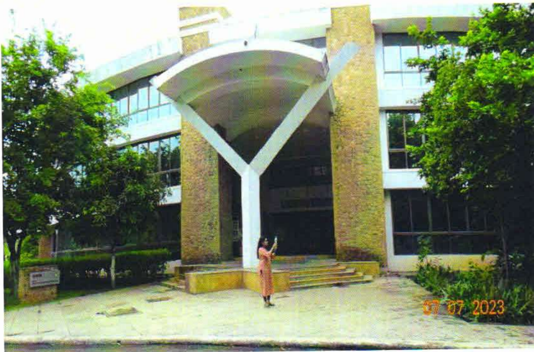
Photo No. 20: Noise Monitoring near DG set
