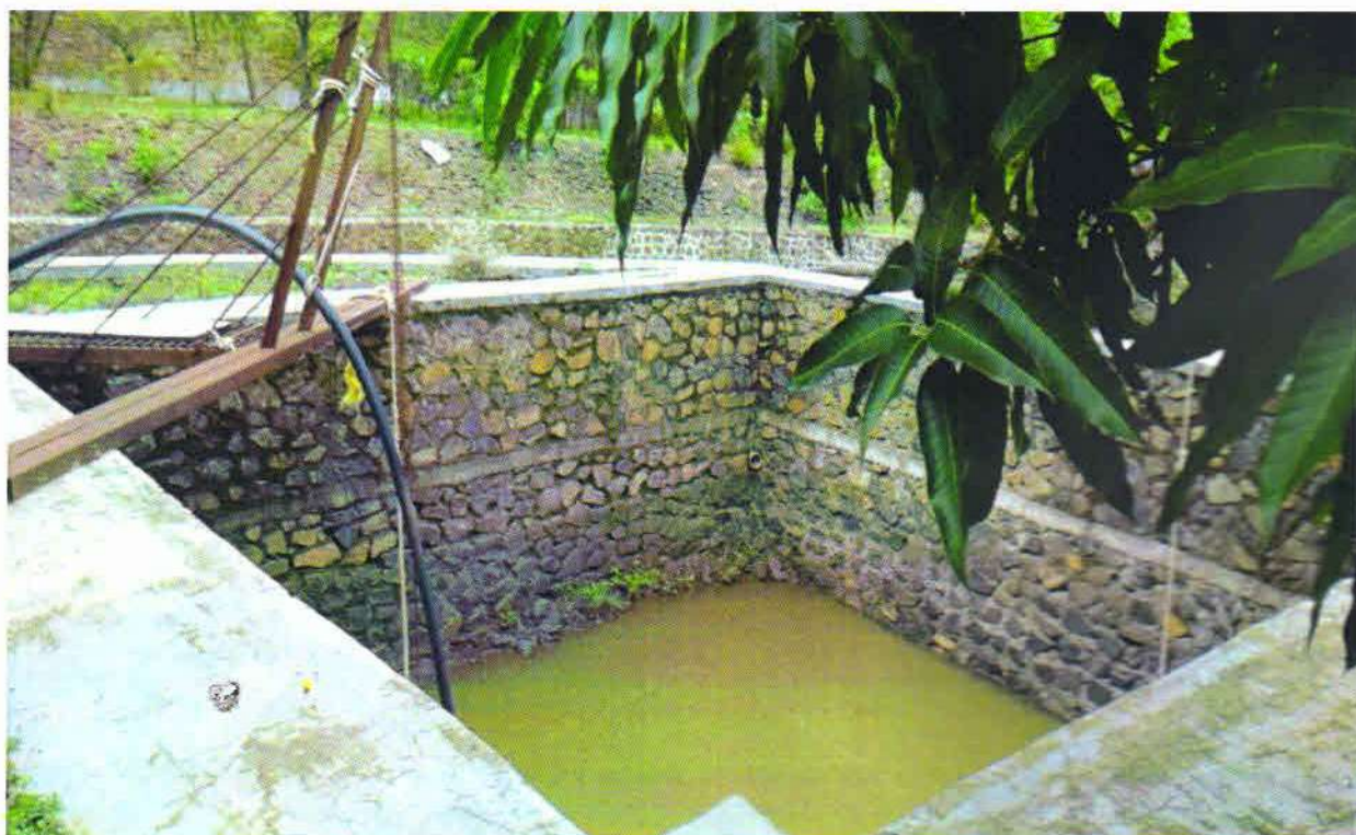
Photo No. 23: Storage tank facility
